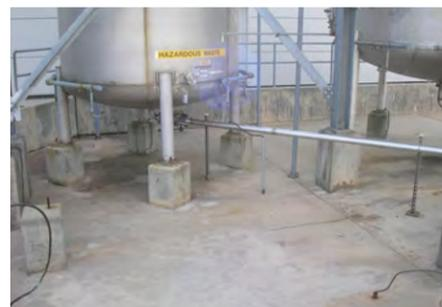
Figure 9. Fixed tanks located within a secondary containment dike comprised of a bottom pad and walls that are designed and constructed to hold spills.
