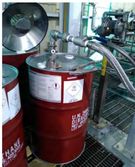
Figure 3. Typical setup for transferring chemicals from a drum to a chemical process. Note the use of an appropriate drum pump, proper bonding and grounding, and secondary containment below the grate.
