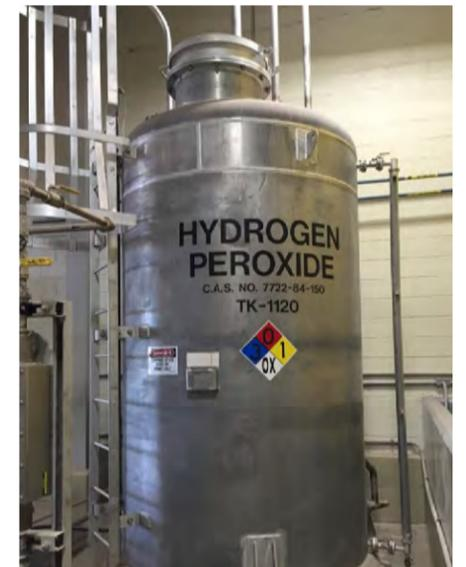
Figure 2. Bulk storage of a chemical in a fixed tank with a hard piped conveyance system and a visual tank level indicating gauge on the right side of the tank.
